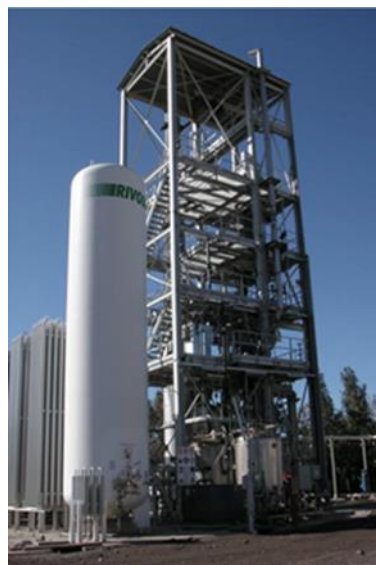
Fig. 3.6 Left - Basic principle of updraft fix-bed gasifier process, Right - Società Tecnologie Avanzate Low Carbon SpA 5 MW biomass gasification (TRL 7-8) [43]
